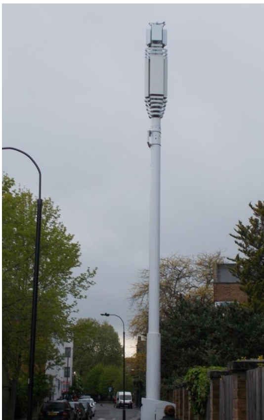
Pic: A similar mast in Farm Lane; bulky cabinets not shown.
